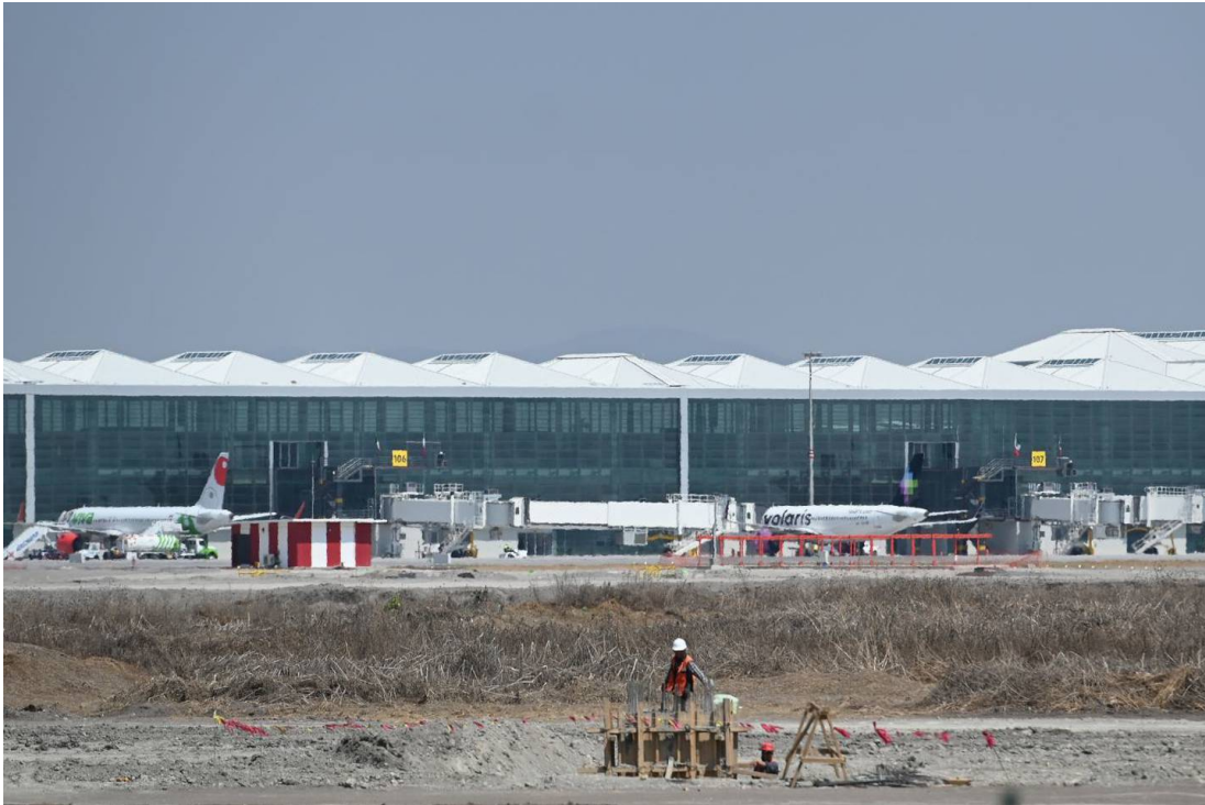
View of the Felipe Ángeles International Airport - AIFA - State of Mexico / Photo Cuartoscuro, March 2022.
